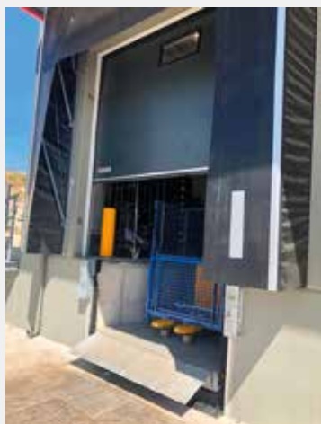
Lifting table with folding half-lip.
